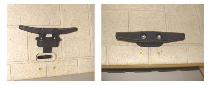
2. Install nylon plate over the bolts sticking through into the channel on the dock section. Place washer and nylock nut onto the bolts and tighten securely. The cleat is now ready for use.
