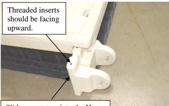
Slide connectors into the H channel on the dock.
