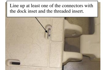
Secure at least one connector with a  $3/8 \ge 2$ " bolt, lock washer and flat washer. It may not be possible to secure both connectors.
