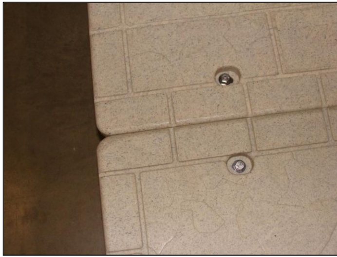
H-Beam Bolted into Dock Sections
