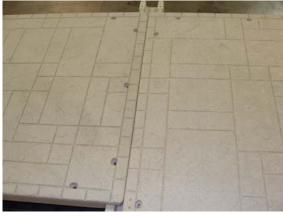
L-Shape with H-Beams sliding into position. H-Beams will not be visible when fully positioned Top view showing alignment of holes and H-Beams sliding into position
