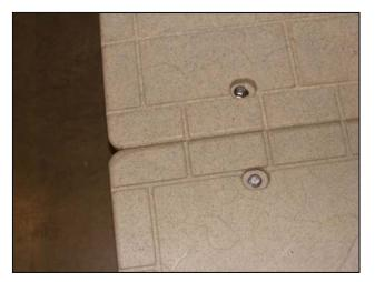
H-Beam Bolted into Dock Sections
